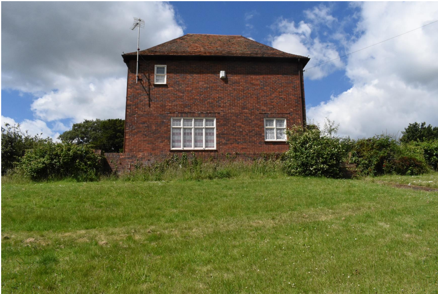
Plate 9: View of the north eastern end of the house and retaining wall, scale 1m (facing W)
