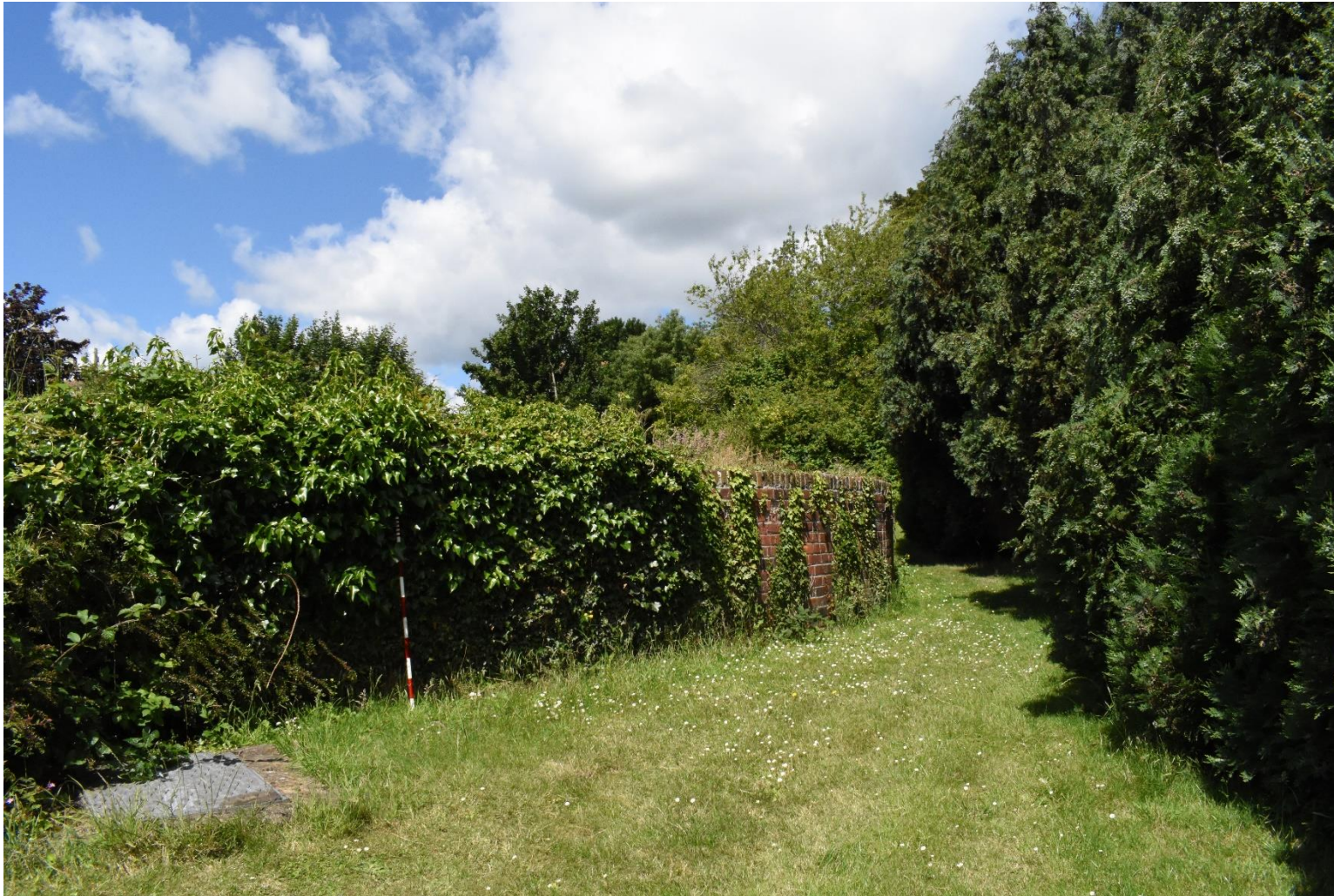
Plate 8: View of the retaining wall, north western side, scale 1m (facing NW)
