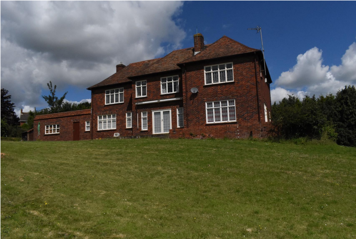
Plate 10: View of the rear of the house, scale 1m (facing NW)
